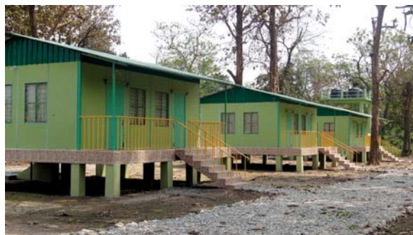
Eco-tourism Camping Facility at Nimati
