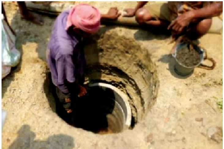
Digging of Ring Well
