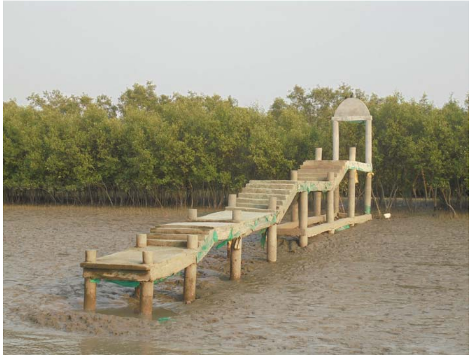
Construction of Jetty, Sundarban
