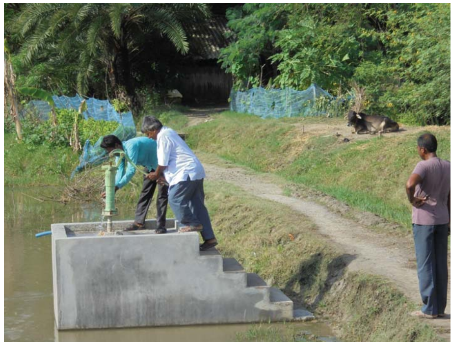
Sinking of Deep Tube Well, Sundarban
